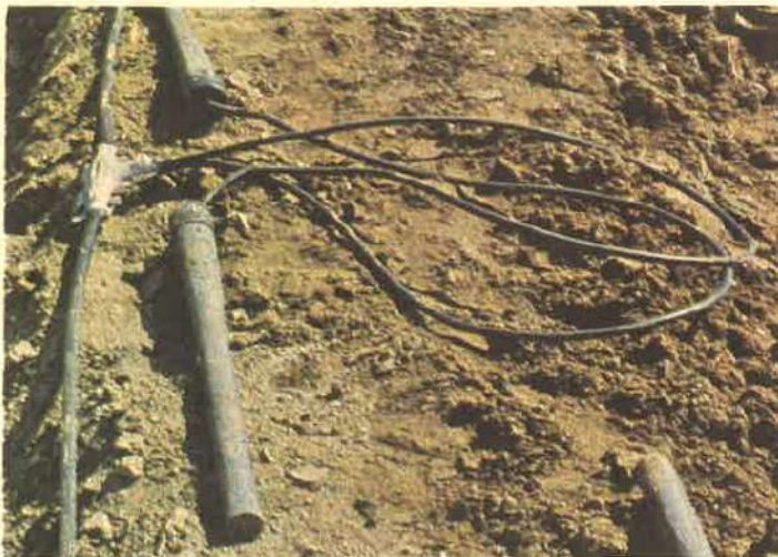
A Stage in anode bed construction, anodes are laid horizontally in a backfill of coke breeze
