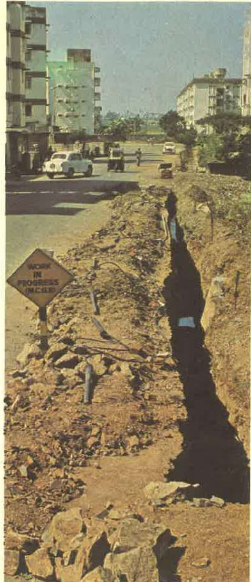
Anode Bed Installation in Urbanised area
