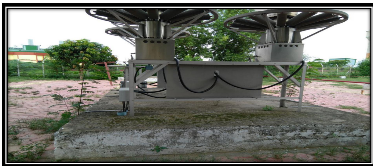
FIGURE 2: TEG SYSTEM WITH MOUNTING STRUCTURE
