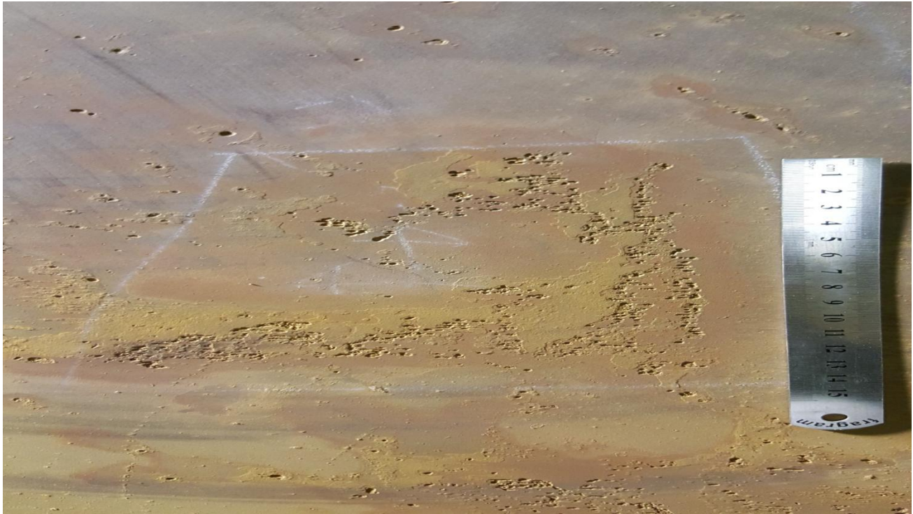
Figure 5: Affected Area on the Bottom Plate of Tanks (Pit Density)
