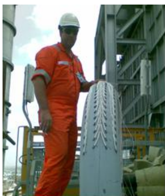
Fig 2: An FSM sensing pin matrix being installed on a high temperature bend in a refinery, India (left), FSMLog instrument (right)
