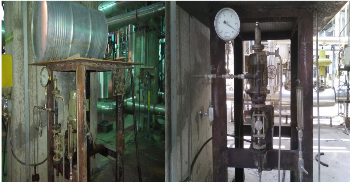
Figure 5: Newly-installed Neutralizer Dosing Pump.
