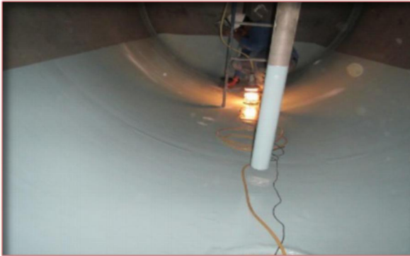
Figure 3: View of Protective Coating application on the inside of the Tank [5].
