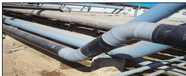
Cold applied thick layer polymeric coating over non-sparking power tool cleaned surface.
