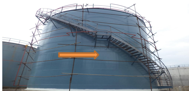
Improved design with hot dip galvanized grating
