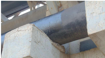
Pipes without corrosion pads
