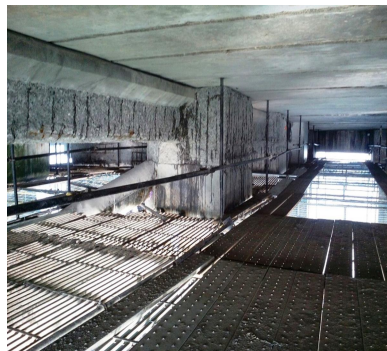
Concrete Corrosion & refurbishment project – Underneath Jetty surface
