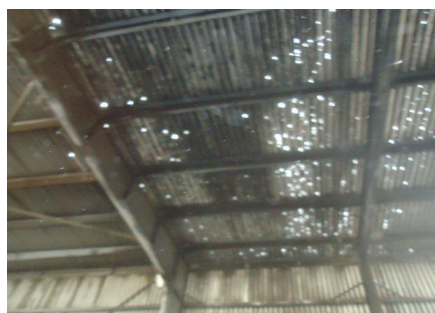
Fertilizers spillage over roof sheet & subsequent corrosion & perforation in AL & Galvalume sheet.
