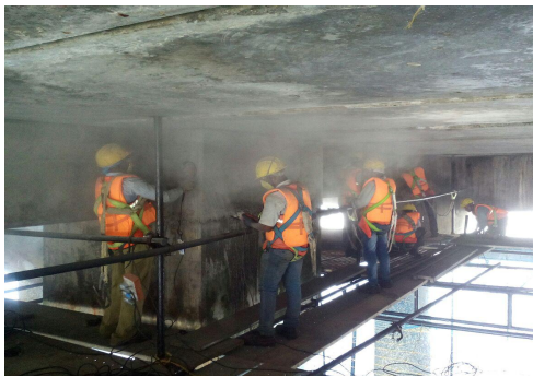
Concrete Corrosion & refurbishment project – Underneath Jetty surface
