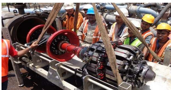
Photograph during launching of MFL intelligent pig in 24" line
