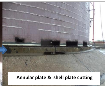
Annular plate & shell plate cutting
