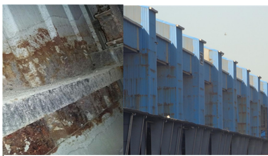
Perforation of Vertical Galvalume sheet
