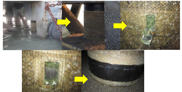
GOOD AFHESION & NO UNDERFILM CORROSION AFTER 3 YEARS OF SEA WATER EXPOSURE
