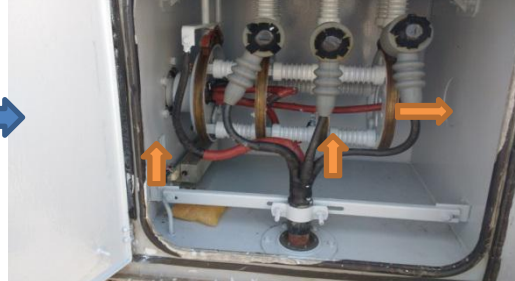
Complete Insulation coating over SS box & Slip ring accessories
