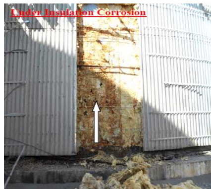
Identification of under insulation corrosion
