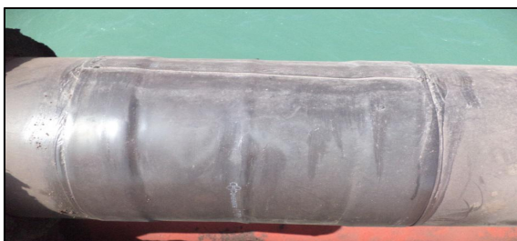
Heat shrink sleeve application in case of Hot work permit availability
