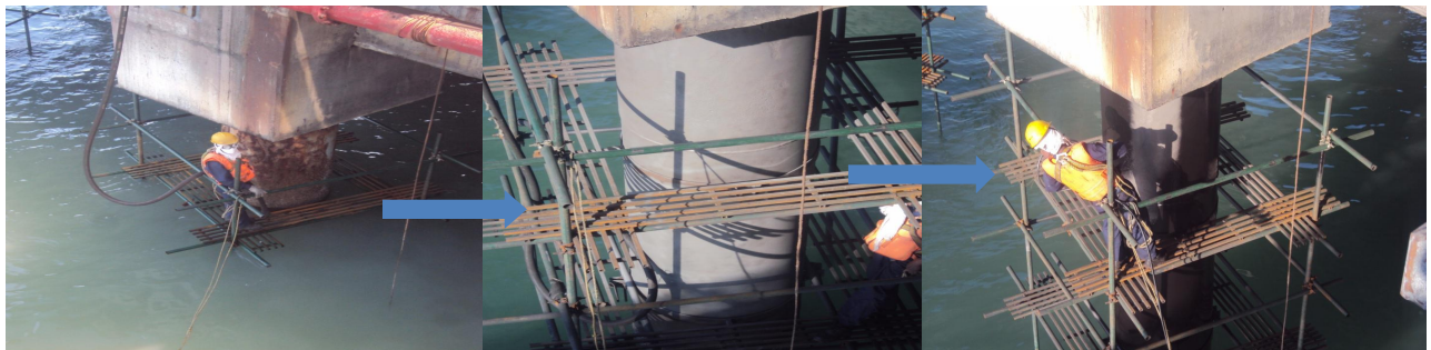
Application of converted epoxy over splash zone area
