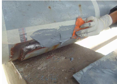
Crevice corrosion of pipes support
