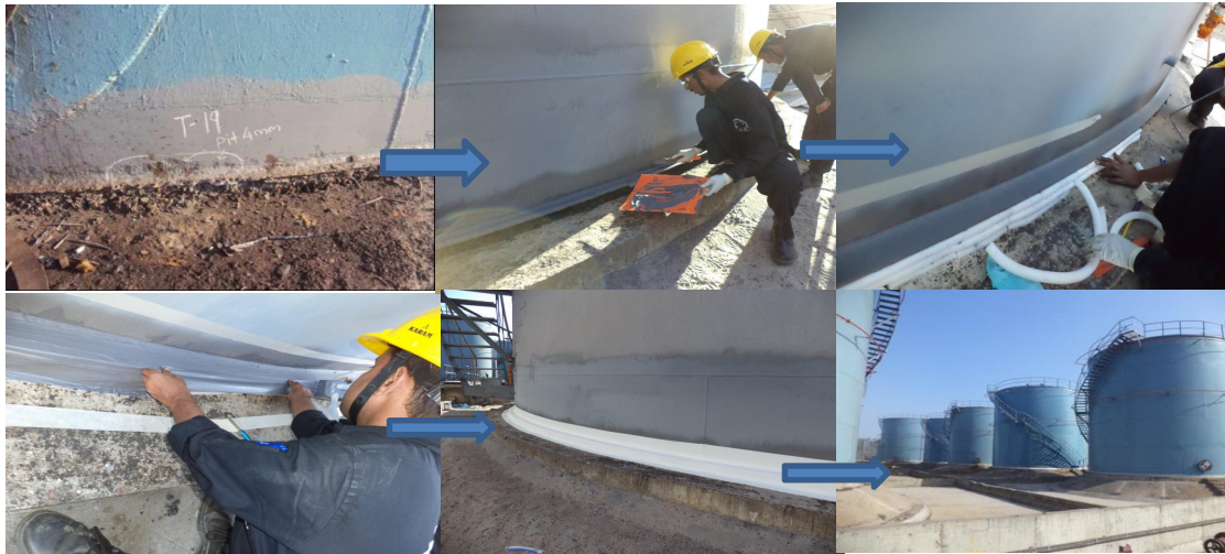
Water based flexible tank bottom seal system implementation over all above ground storage tank
