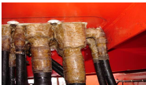
Corrosion protection of hydraulic joints by petrolatum tape
