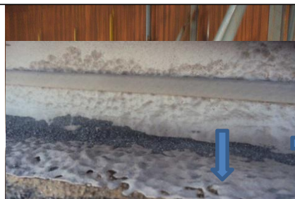
Initial condition - Tank annular plate and bottom plate thinning
