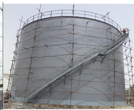
Insulation renewal after tank repair & Blasting coating
