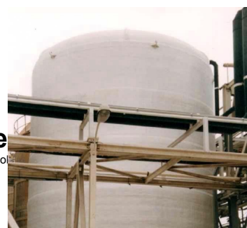
Figure 5: Storage tank for phosphoric acid (max 30%) sulfuric acid (40g/L), and some hydrofluoric acid (2%) 7.8 m diameter, 10.7 m height, in perfect condition after 9 years of service in Spain.
