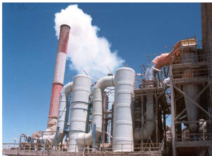
Figure 6: FRP Gas Scrubbing System in Tunisia, 7.5 m height, 2.5 m diameter.
