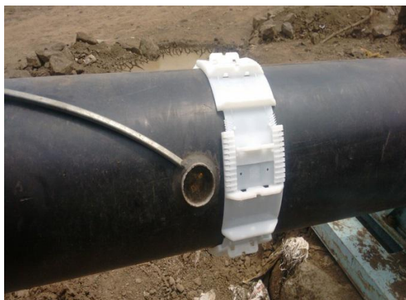
Figure 5: Spacers and Zn ribbon anodes on carrier.
