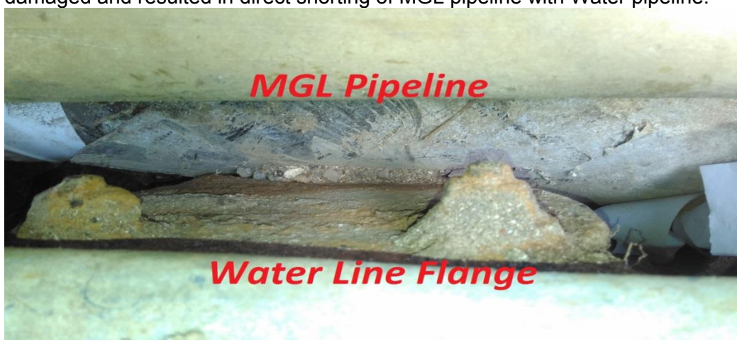
Figure 4: Shorting of MGL Gas Line and Water Line
