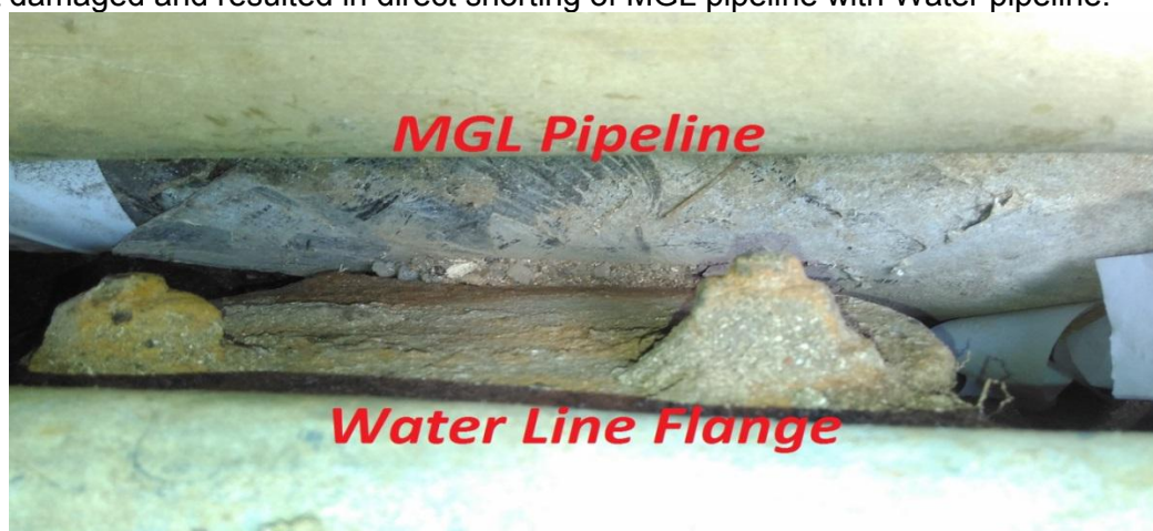
Figure 4: Shorting of MGL Gas Line and Water Line
