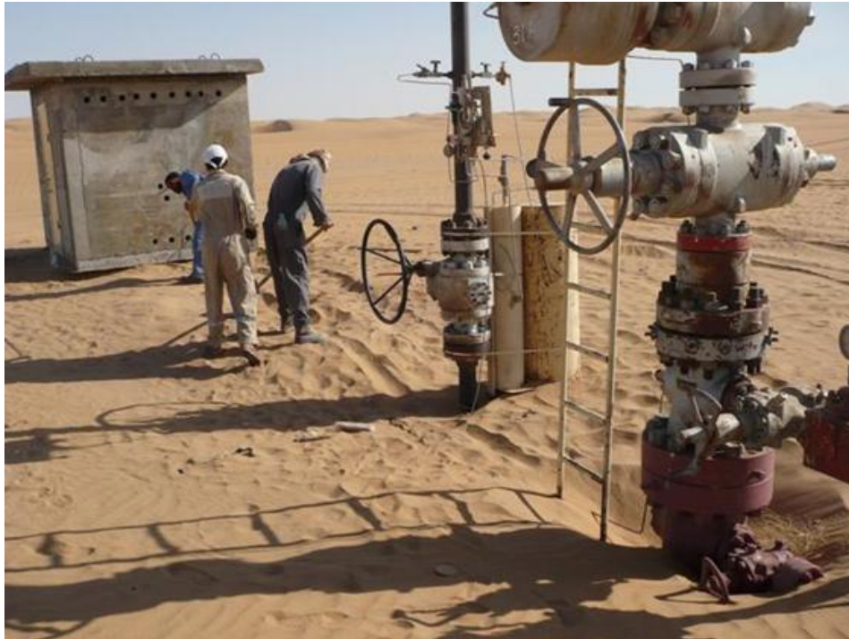
Figure 4: Al-Raja Gas Field Well Casing CP System by TEG.
