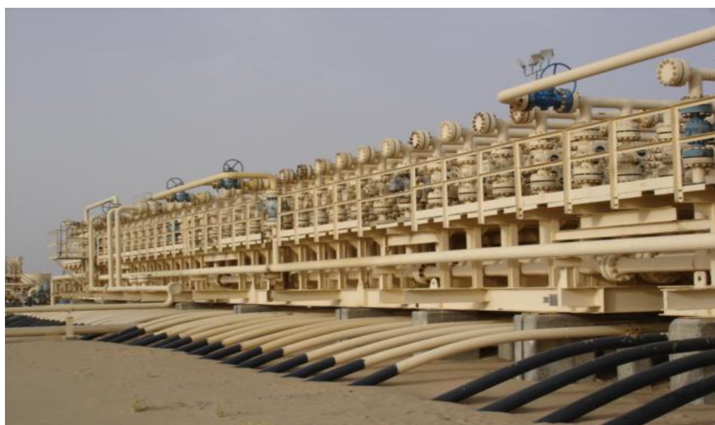
Figure 2: Flow line gathering station
