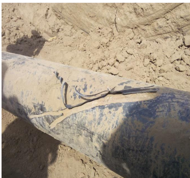
Fig.- 4 Coating & pipe damage at Ch. 617.550 Fig.-5 Coating & pipe damage at Ch. 617.600
