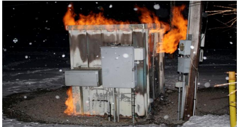
Figure 3. Fire at a regulator station resulting from a fault near unprotected isolation joints
