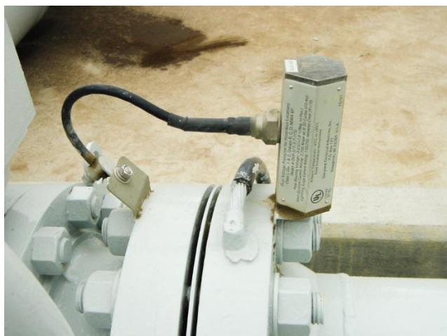
Figure 4. Solid State Over-Voltage Protector
