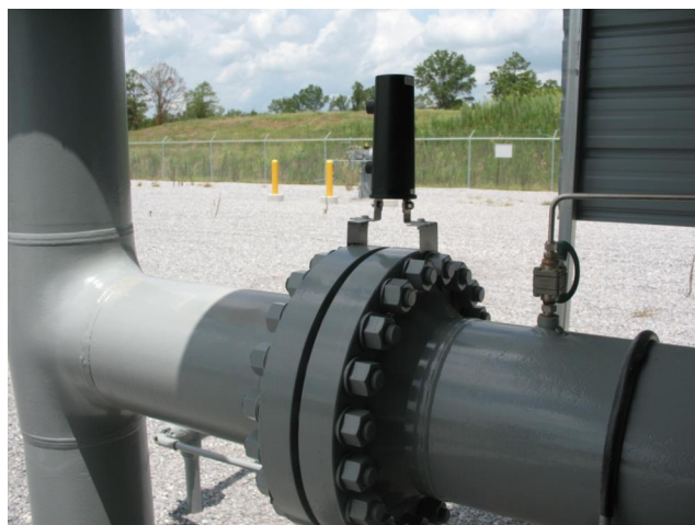
Figure 5. Solid State Decoupler
